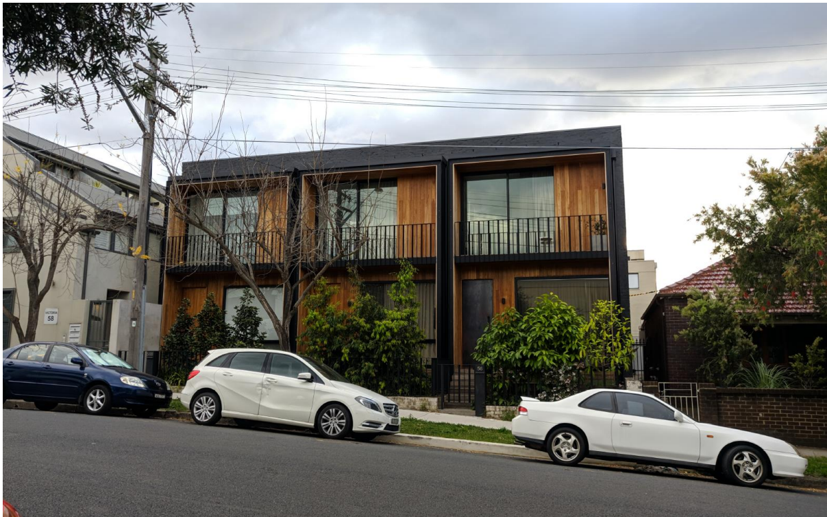
Figure 5: 56, 56A and 56B Victoria Street located to the south of the site, consisting of 3 x attached terrace dwellings within an adaptively reused former warehouse building (2019 photograph taken by Council officer)
